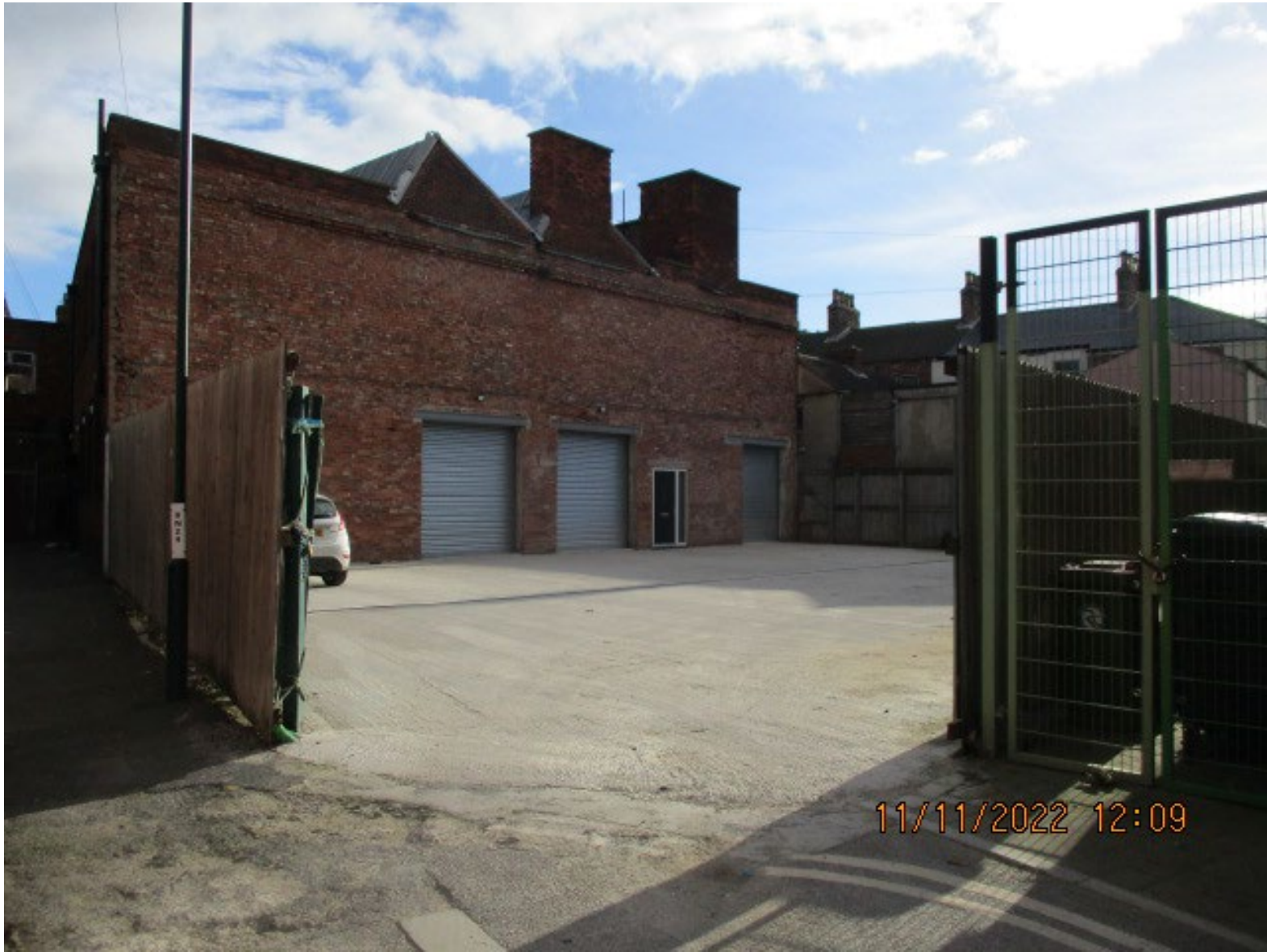
R/2022/0802/FF – Rear of 60 Station Road, Redcar Photos
