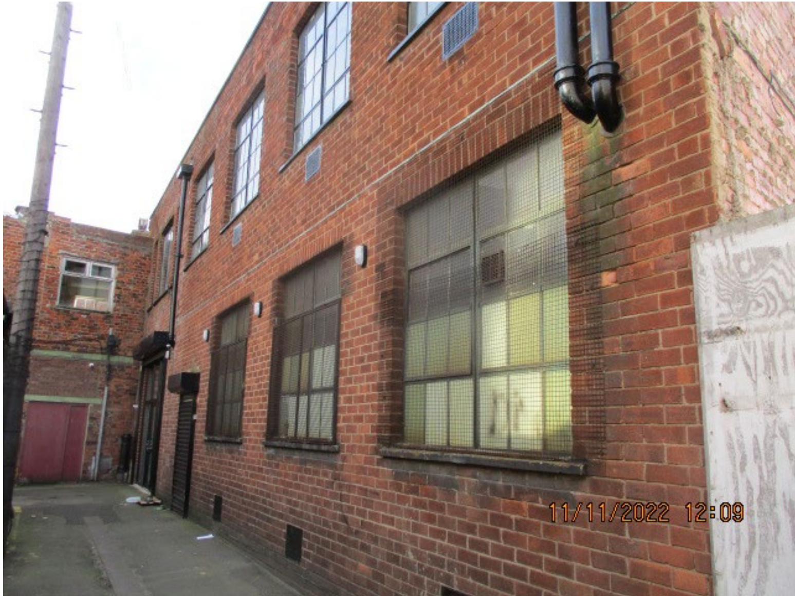
R/2022/0802/FF – Rear of 60 Station Road, Redcar Photos
