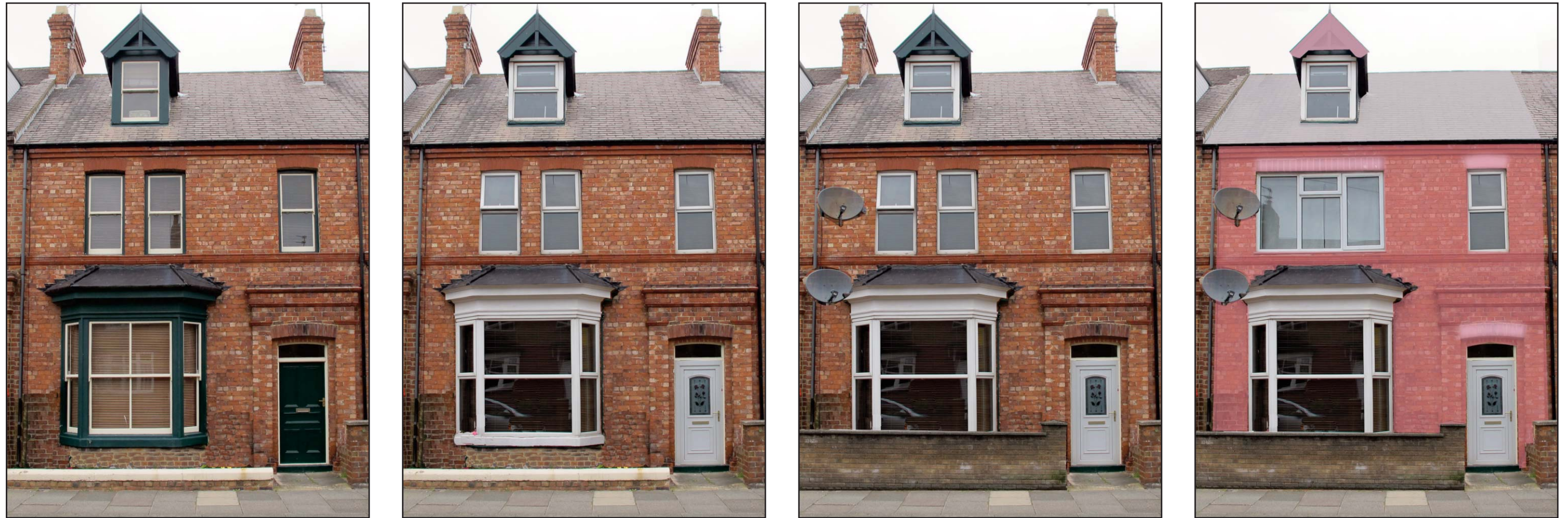
Cumulative unsympathetic and damaging results of alterations*
