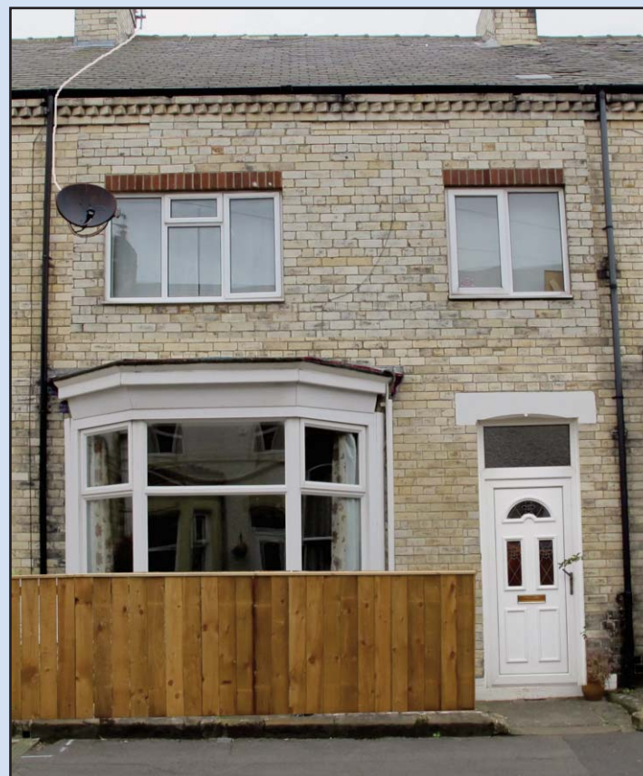
Inappropriate close boarded timber fence*
