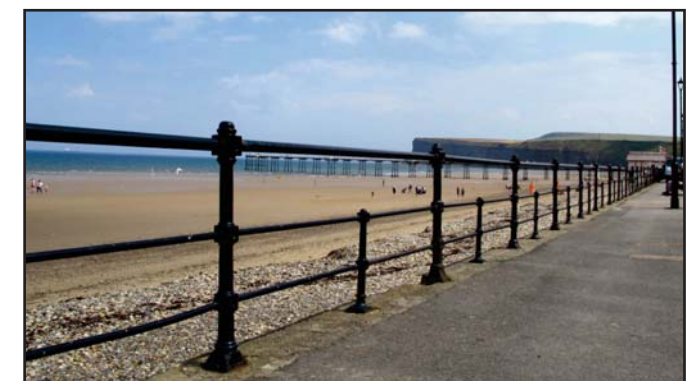
Cast iron railings on the foreshore
