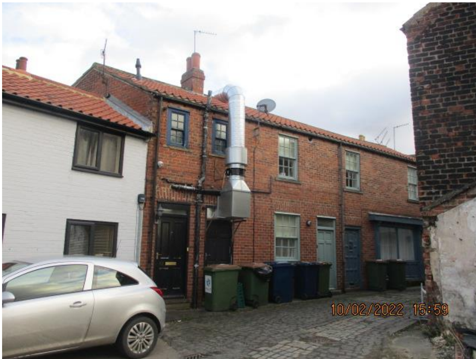
R/2022/0020/CA Badgers, 55 – 57 Church Street, Guisborough Photographs
