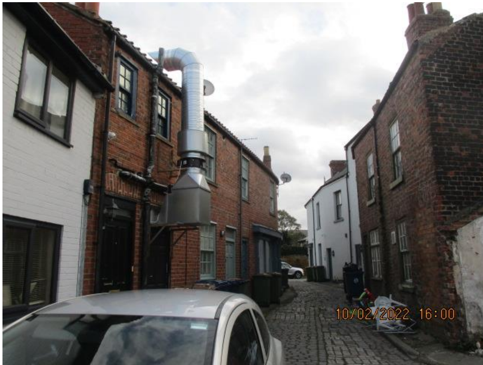
R/2022/0020/CA Badgers, 55 – 57 Church Street, Guisborough Photographs
