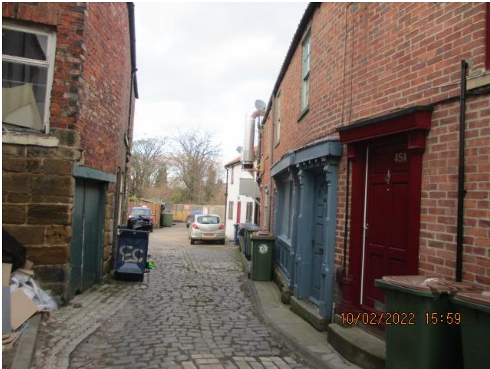
R/2022/0020/CA Badgers, 55 – 57 Church Street, Guisborough Photographs
