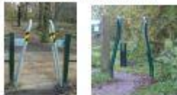
Typical 'A Frame' Barrier Access
