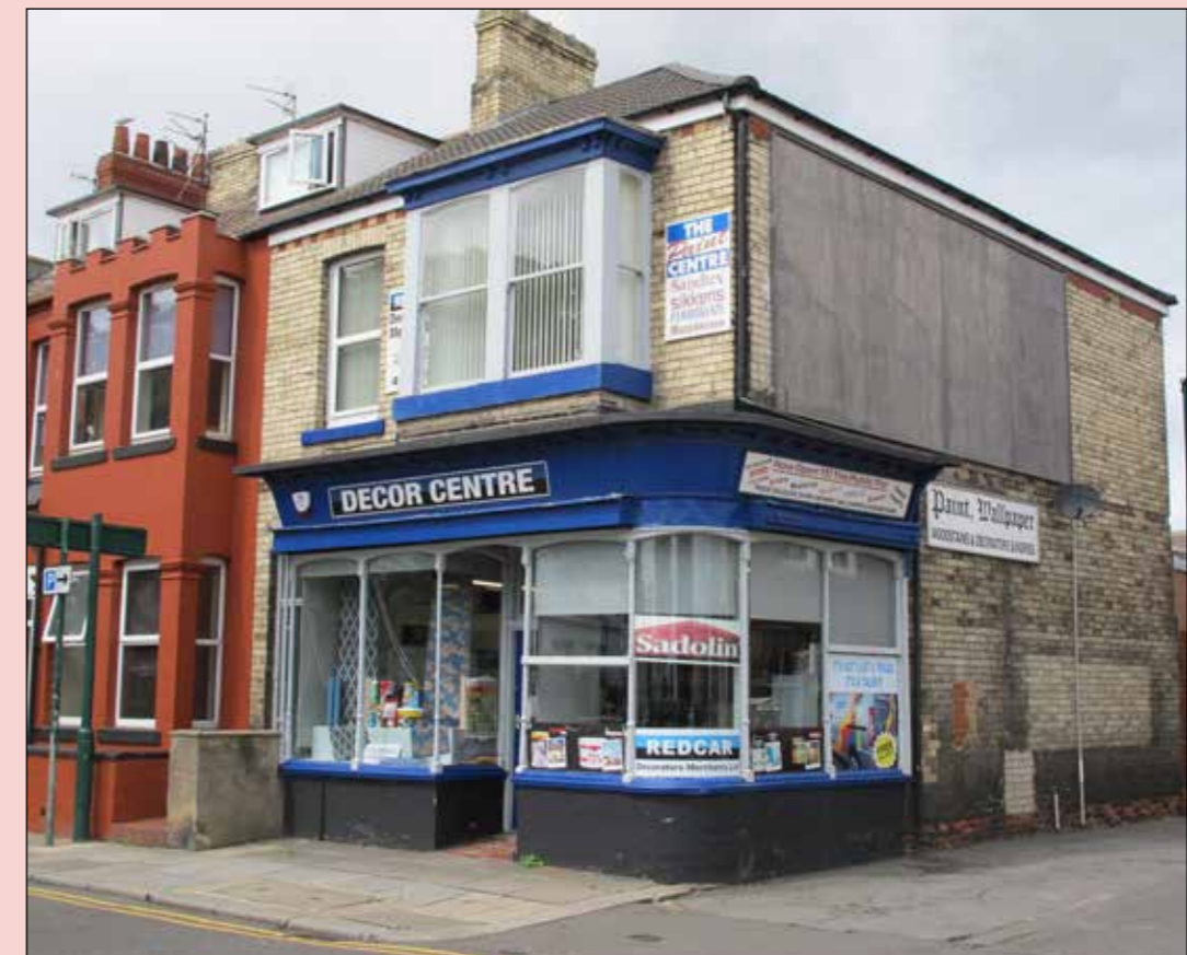
The last remaining historic shopfront in the conservation area, 102 Coatham Road
