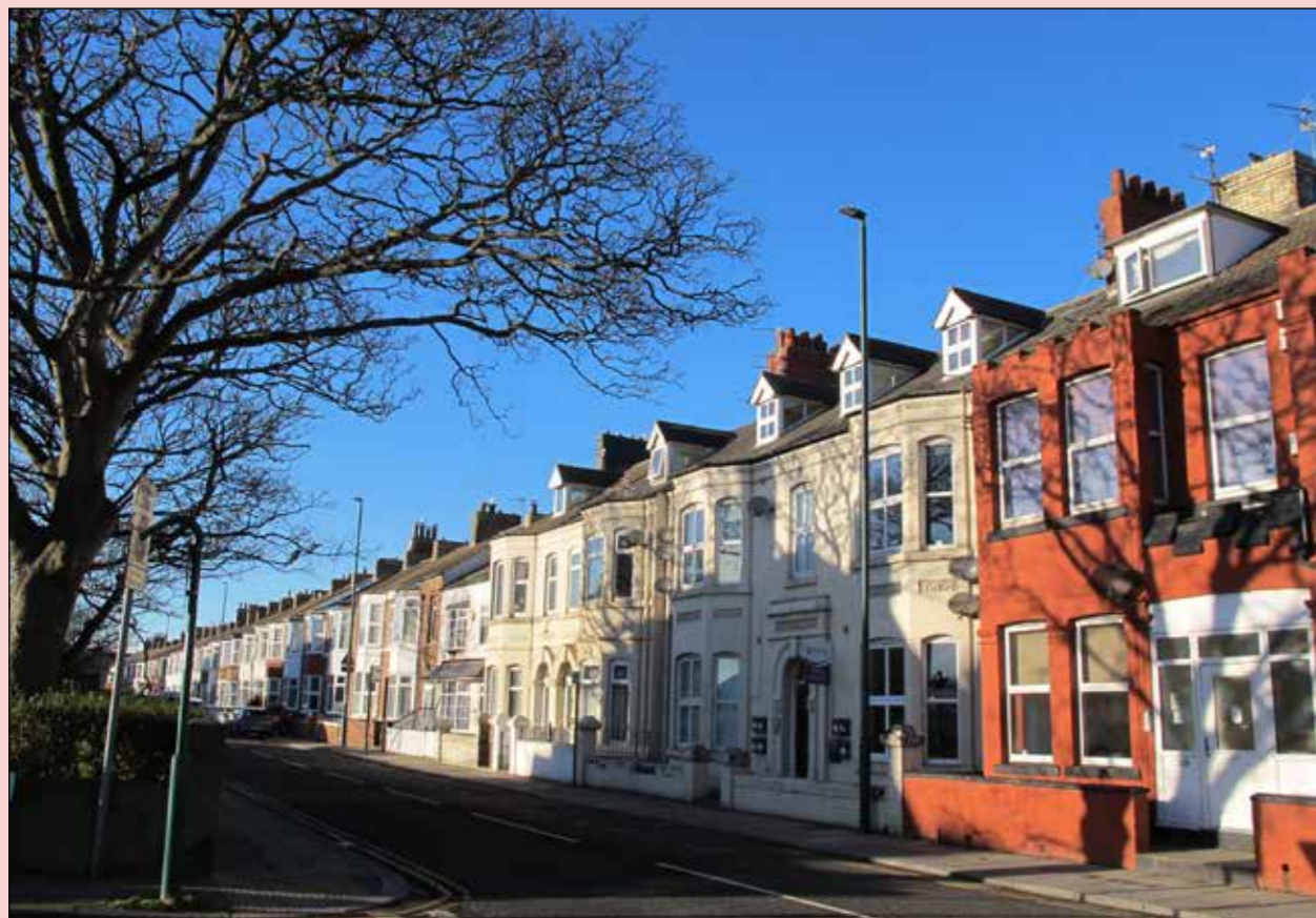
North side of Coatham Road
