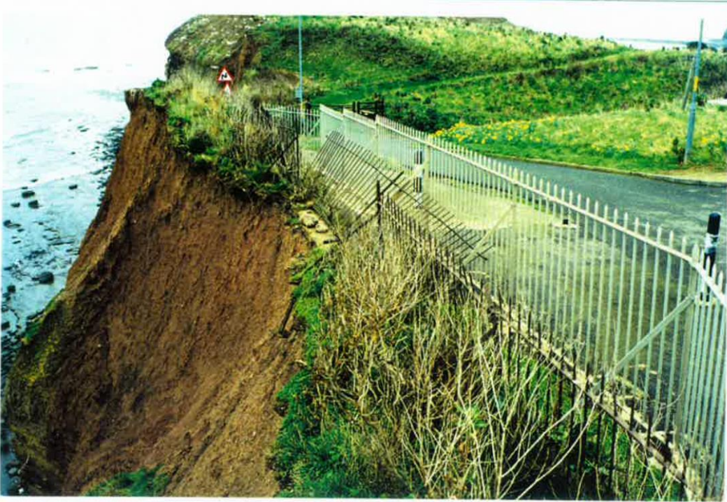
Plate16a The oversteepened glacial till slope at Cowbar Cottages. Note the spalling failure of the glacial till (bottom left hand corner).
