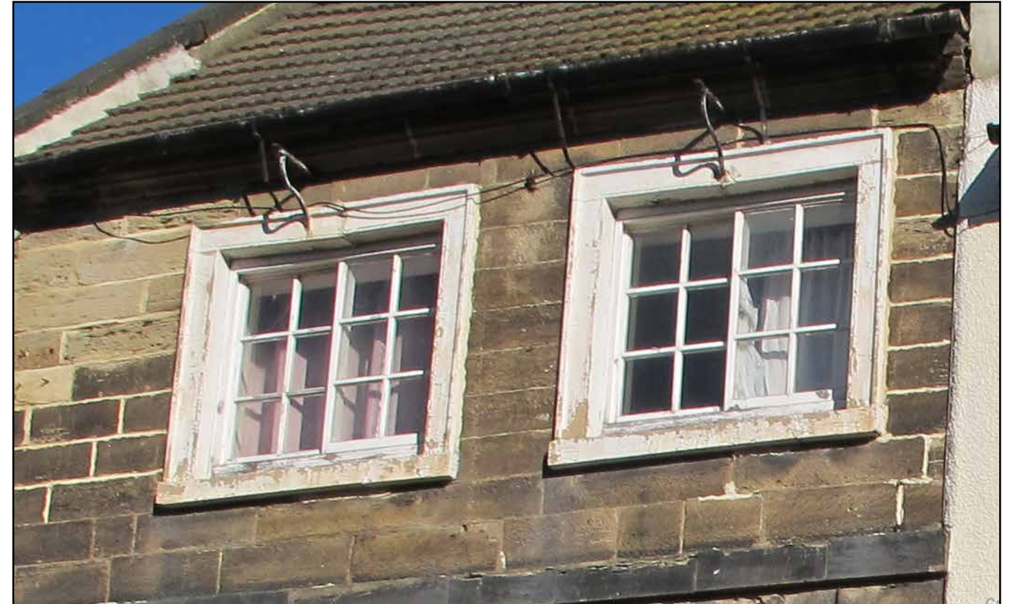
Horizontal sliding sash windows, known as "Yorkshire" sliding sash
