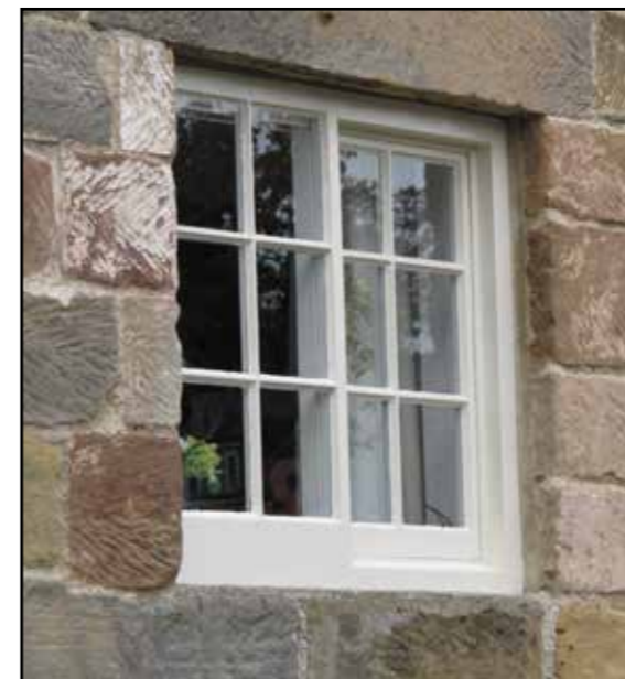
Sliding sash windows in Loftus, both vertical and "Yorkshire" horizontal types. Some are likely to be original pitch pine which if maintained properly can last indefinitely
