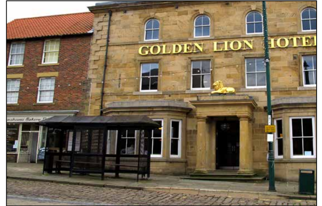
Highway infrastructure obscuring the façade of a key historic building
