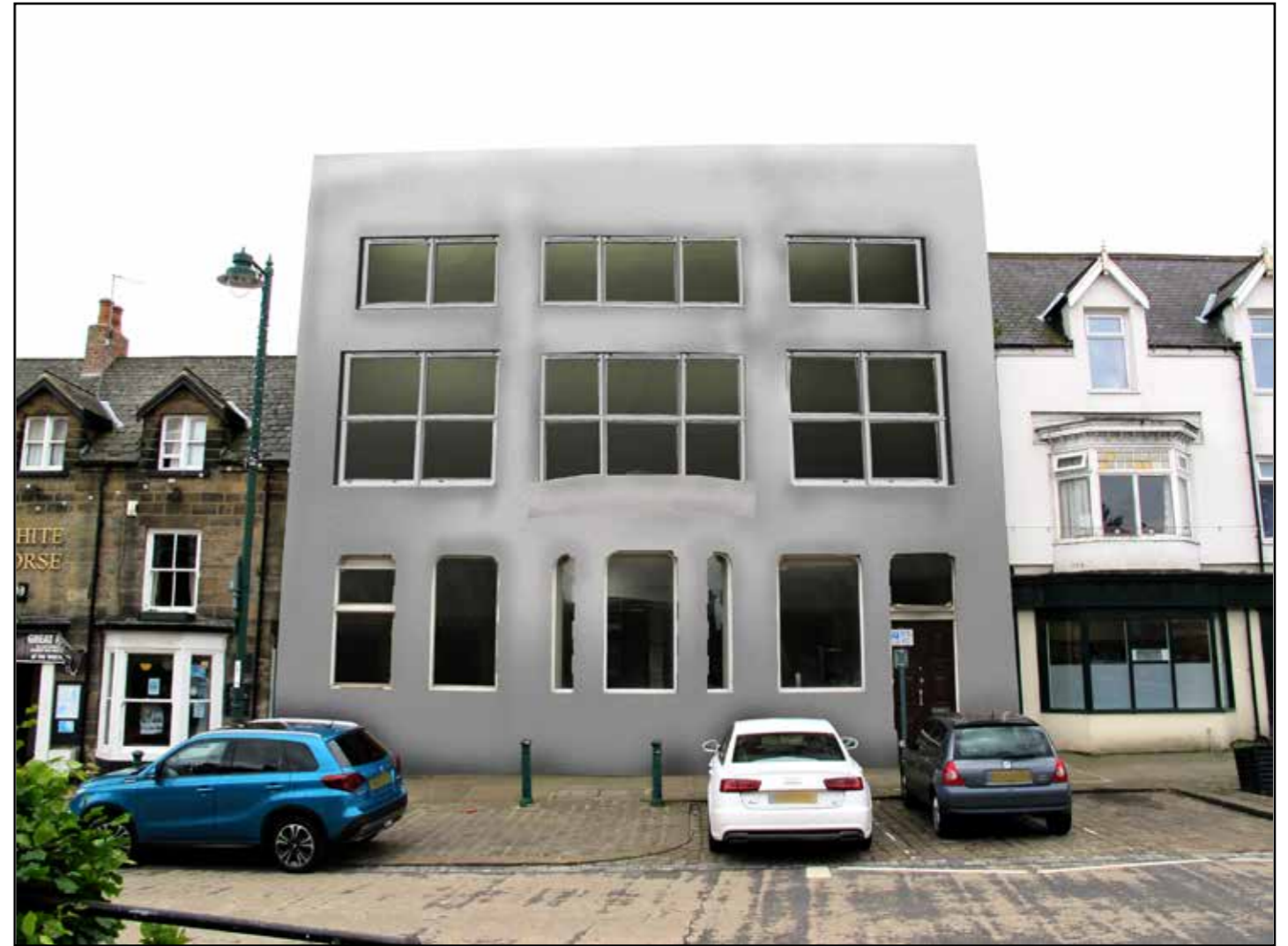
Modified image showing harmful alterations to the façade of a classical building
