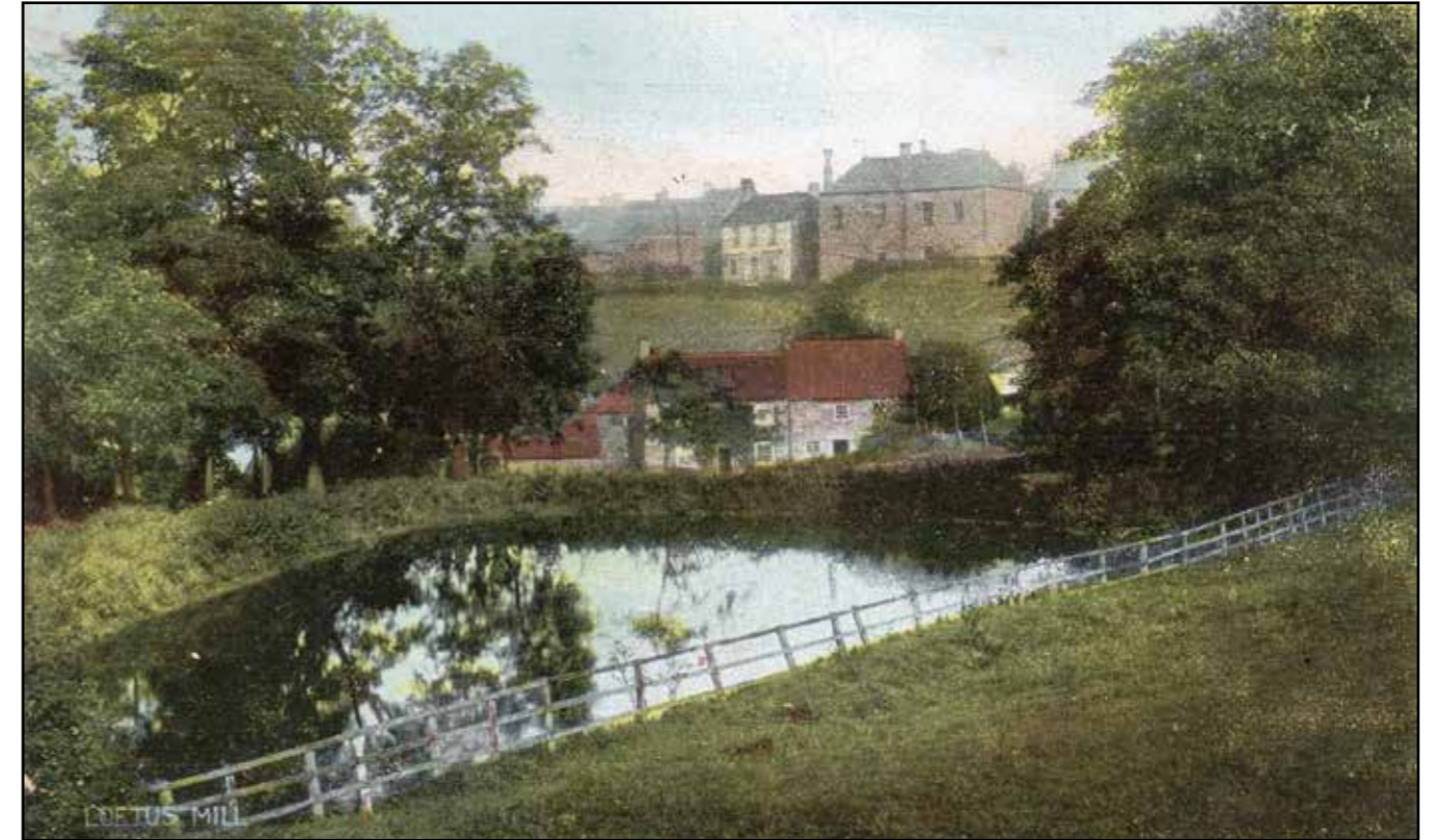
View towards Loftus Mill, now obscured by tree growth
