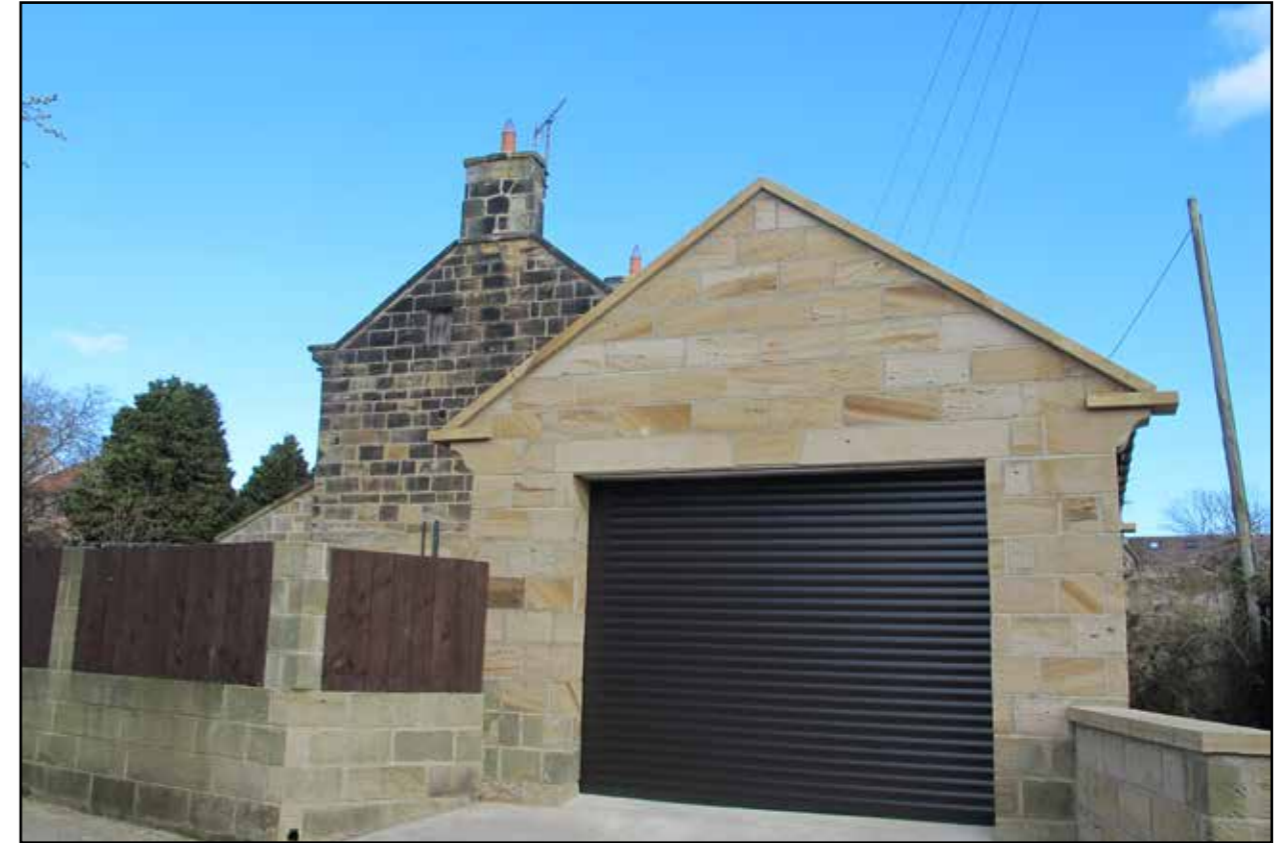
New garage reflecting traditional character and materials
