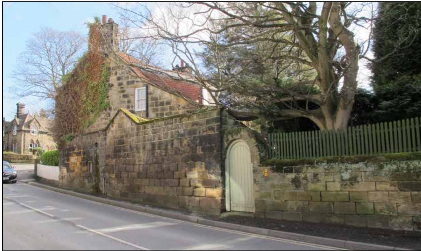
Historic Listed Wall, Jessemine Cottage
