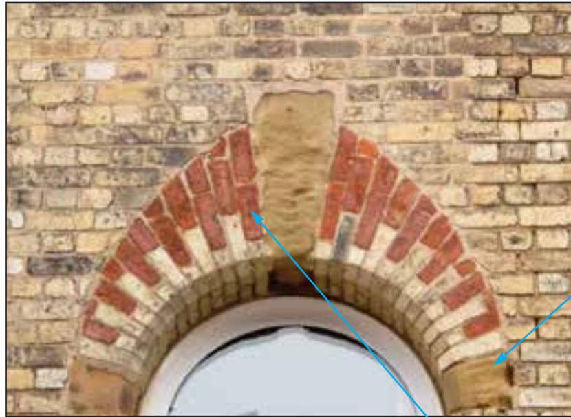
Stone used for bands and dressings around windows and doorways.
