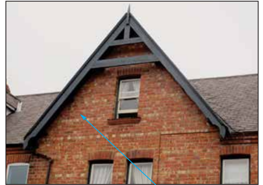
Timber used for windows, barge boards and other decorative details such as the domestic revival inspired houses on the western side of Upleatham St which have a half-timbered appearance.
