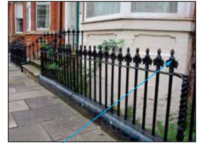
Iron used for front railings.
