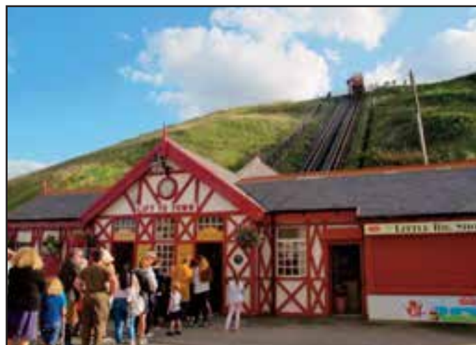
Lower Promenade Buildings
