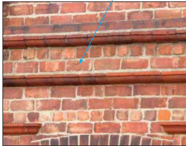
The bricks were laid in a range of different bonds, including 'Flemish' and 'English Garden Wall'.
