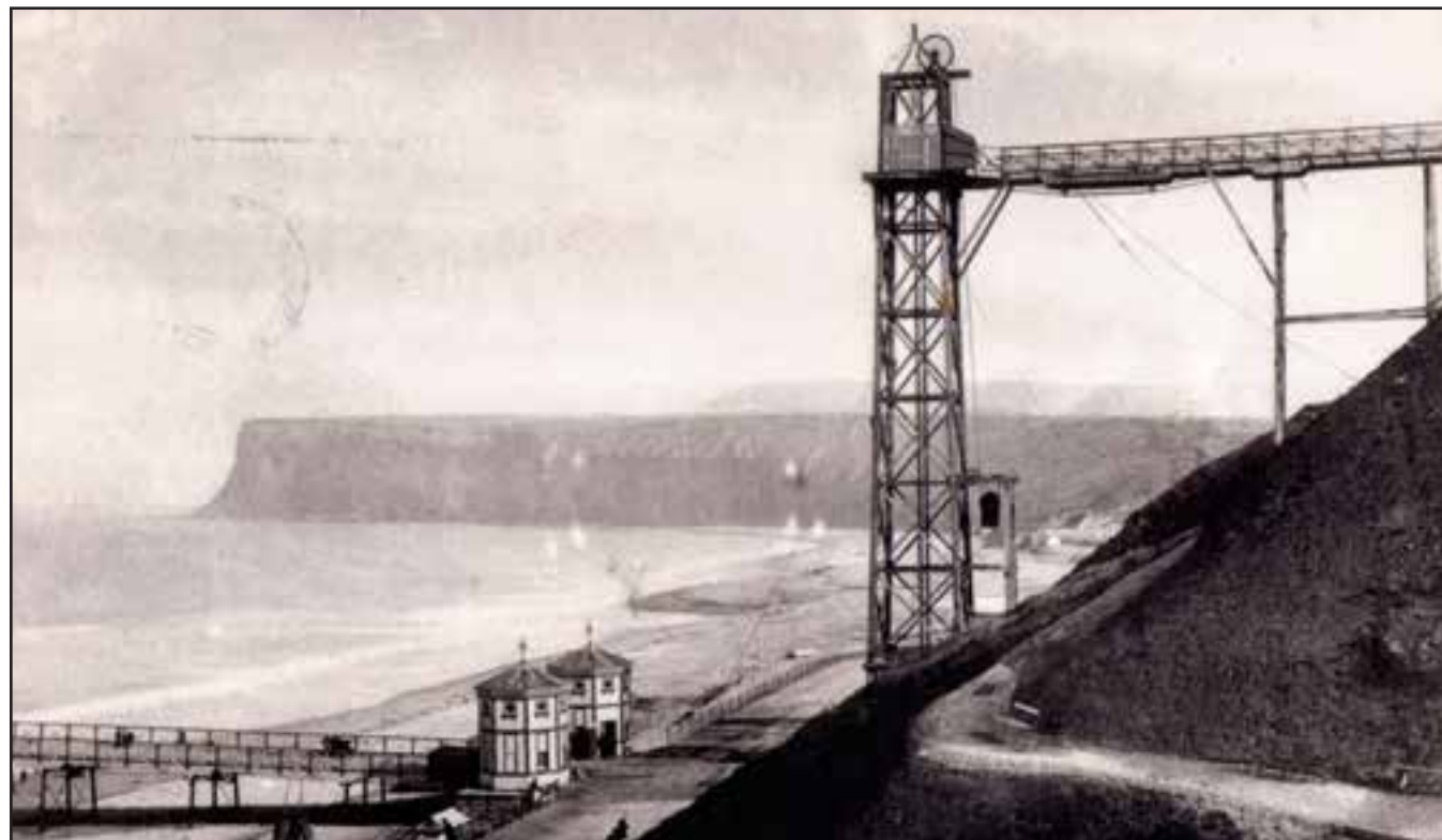
Saltburn's original cliff lift, a hoist mechanism dismantled in 1883
