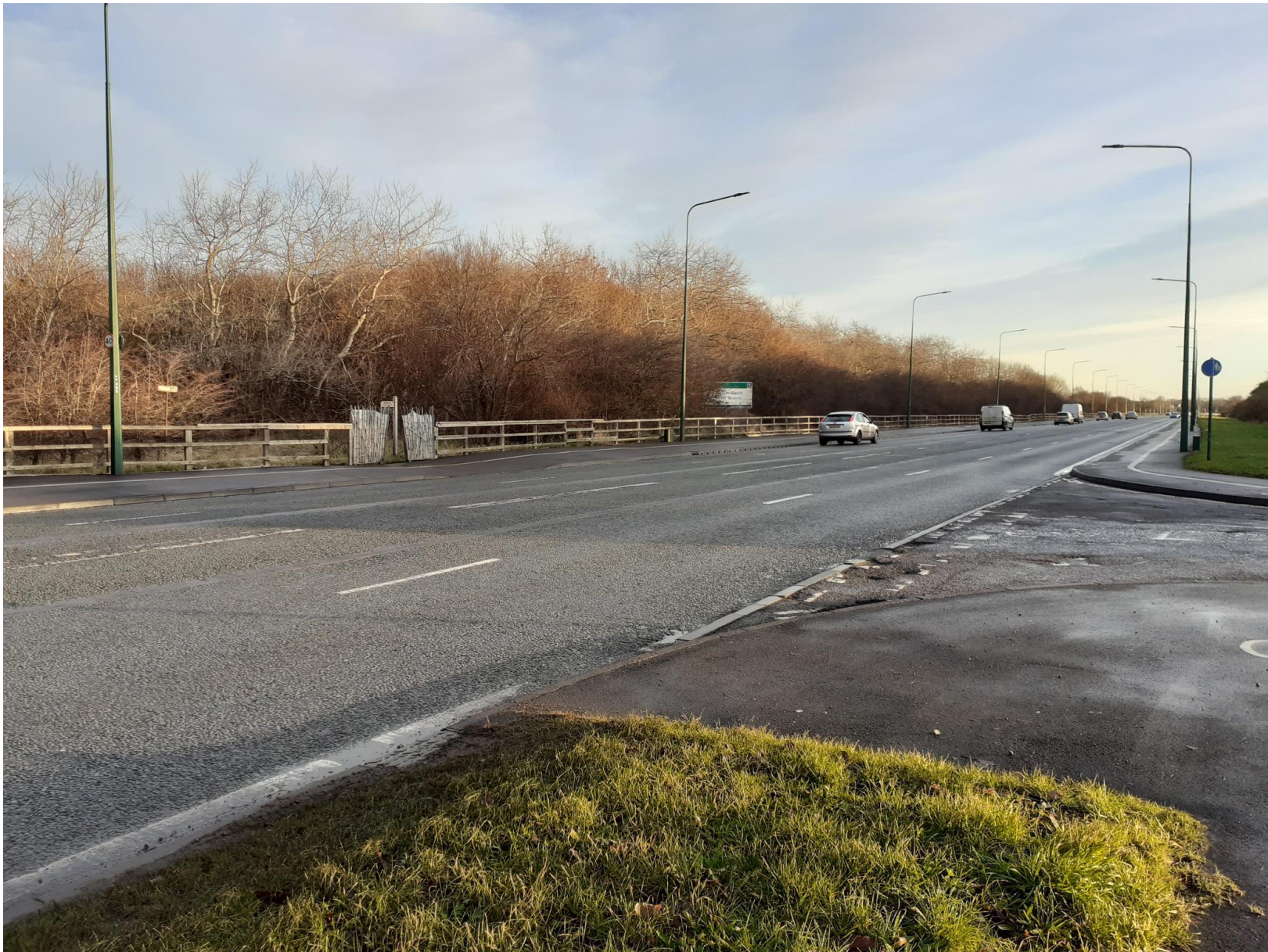
R/2022/0816/FFM - North of Trunk Road Photos
