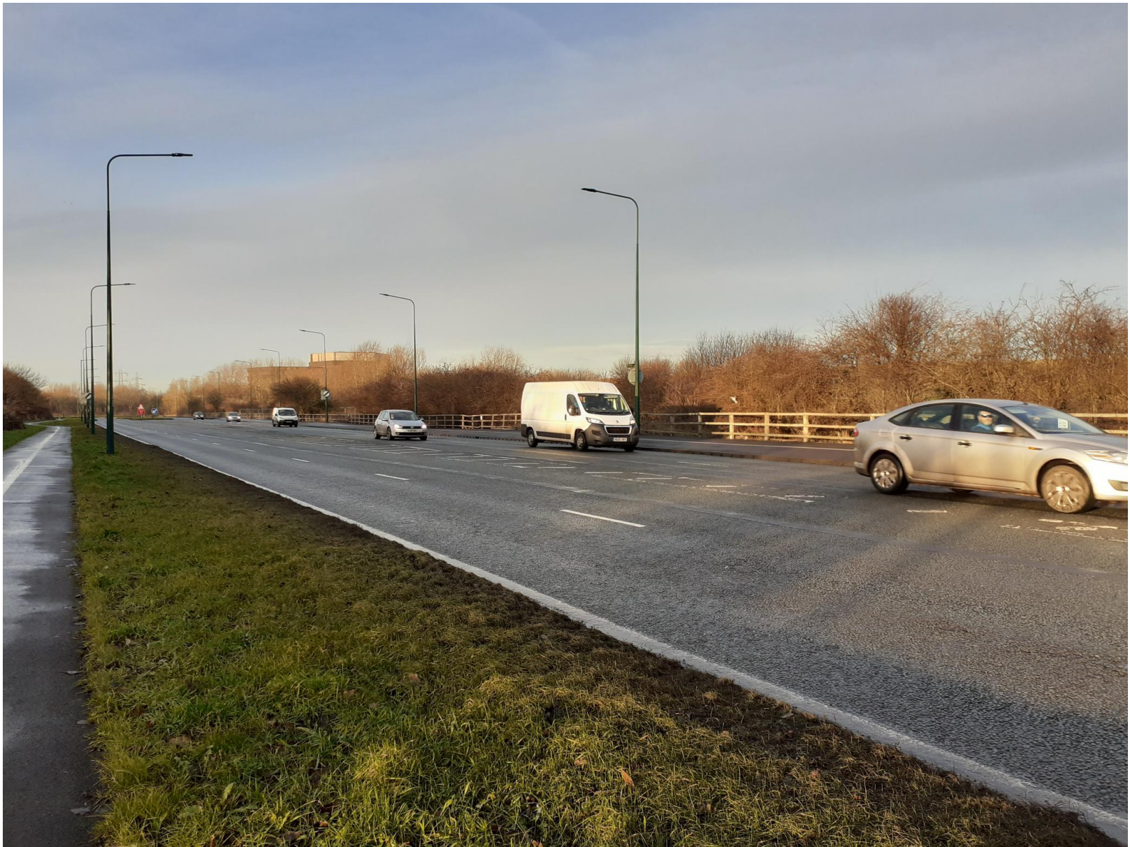
R/2022/0816/FFM - North of Trunk Road Photos
