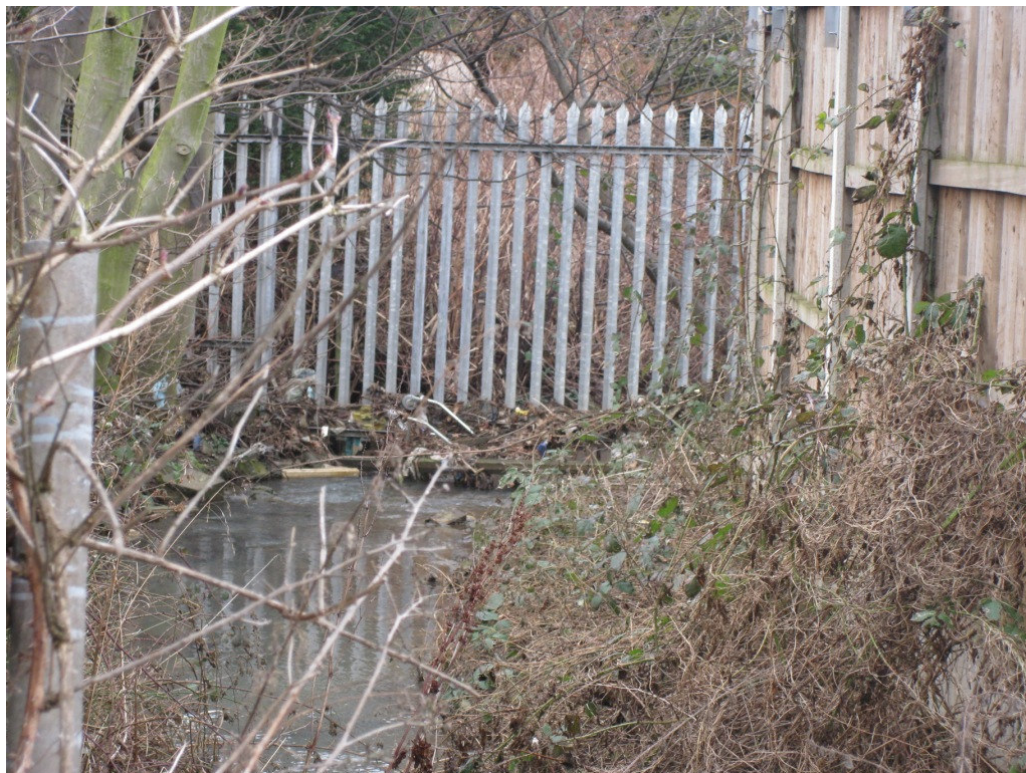
Figure 22 - Fence across a watercourse in Eston
