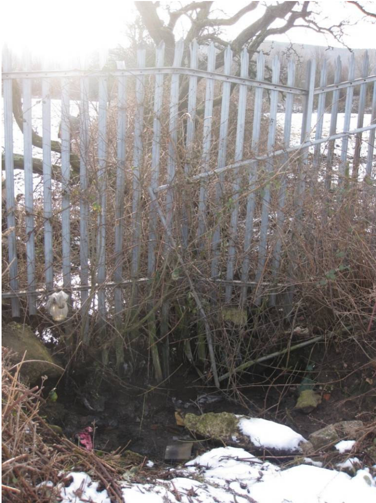
Figure 12 - Looking u/s at a field drain as it enters Guisborough
