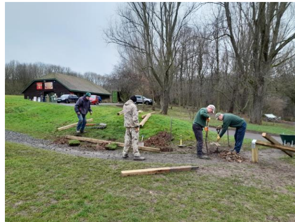
Fencing at Flatts Lane
