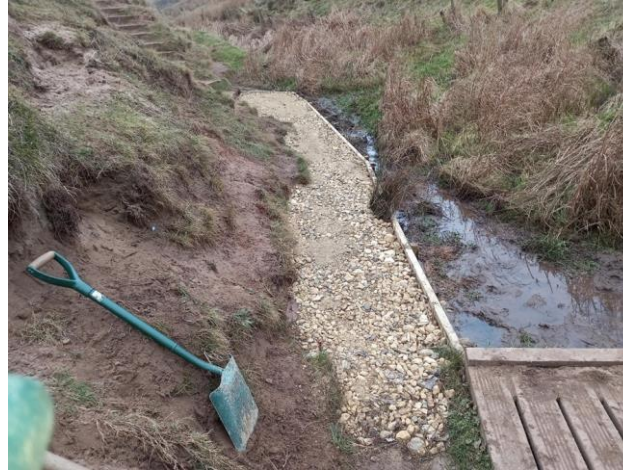
PROW path repairs
