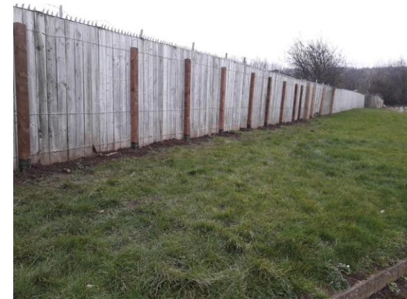
Bankfield Allotments Repairs
