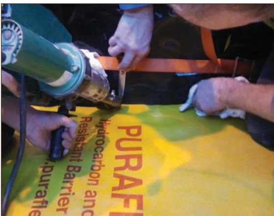
Figure A4.29 Extrusion welding technique (courtesy Industrial Textiles & Plastics Ltd)
