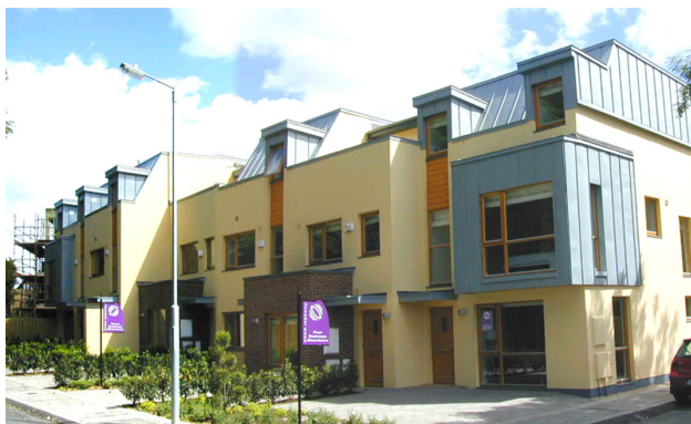
Fig 73. Contemporary modern terrace at Malahide, north of Dublin. Mansard roofs give a large volume of internal space to the attic storey of these developments. Roof terraces at the rear supplement front and back gardens.
