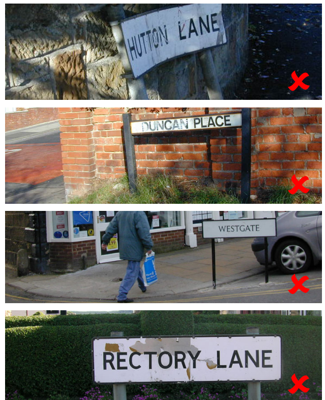
Fig 116. Pole mounted examples where adjacent walls present alternative locations. To install examples such as these is to increase the risk of vandalism to to commit to unnecessary and ongoing maintenance and replacement
