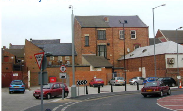
Fig 143. A plethora of signage and infrastructure, installed without consideration of negative cumulative impact.
