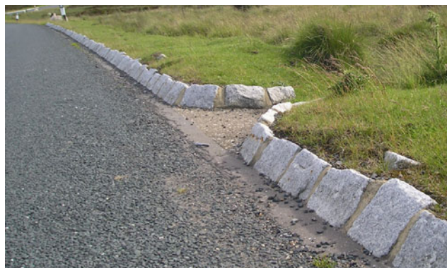
Fig.150. Road edging design within the national park. Durable materials in sympathy with their rugged context.
