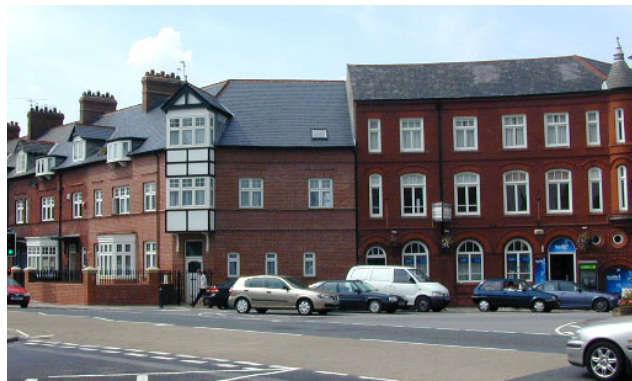
Fig 15. The completed infill of Fig 14, unifying two different facades and turning the corner with a point of interest via a projecting bay, achieving quality and response to context and adding significantly to the streetscene.
