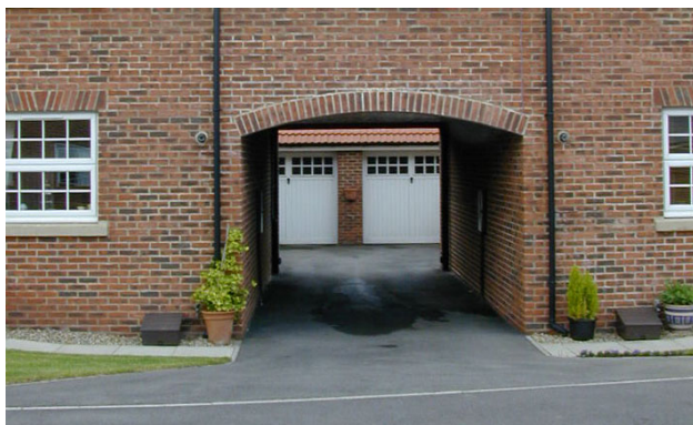
Fig 64. In curtilage parking discretely located through carriage arch. Accidental trespass is highly unlikely here.
