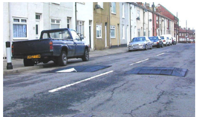
Fig 101. Crude 'bolted on' traffic calming which should be designed-out through improved layout in new schemes.
