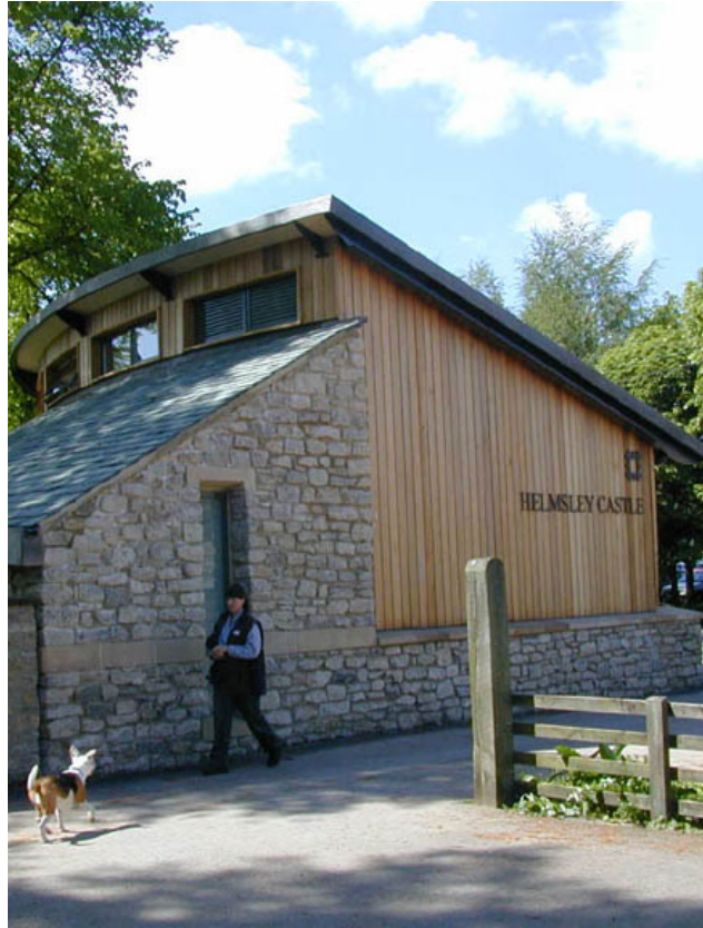
Fig 66. Helmsley: Contemporary design using traditional materials sympathetic to context.
