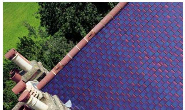
Fig 81. Photovoltaic 'Solar roof tiles' contributing to meeting the energy needs of a terraced house. (Image Solar Century Ltd)
