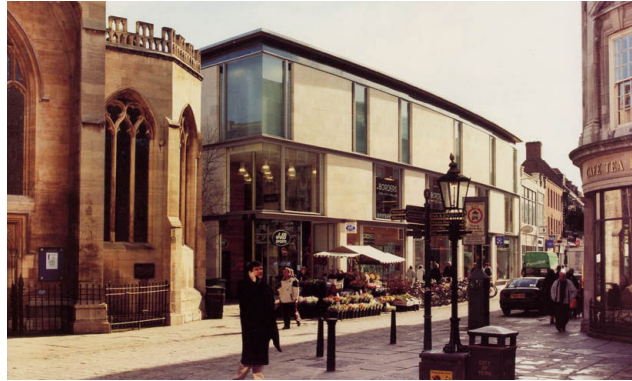
Fig 19. New retail development, York. Respects the building line and scale of its neighbours without imitation.
