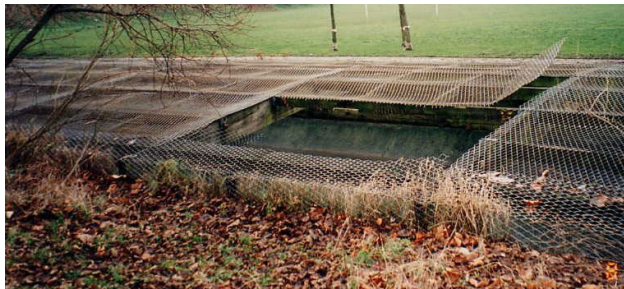
Fig 161-2. The Cong Burn, Chester-le-Street, was constrained in a concrete culvert, squandering a valuable landscape resource. A misguided health and safety mentality had created a steep sided, mesh covered health hazard.
