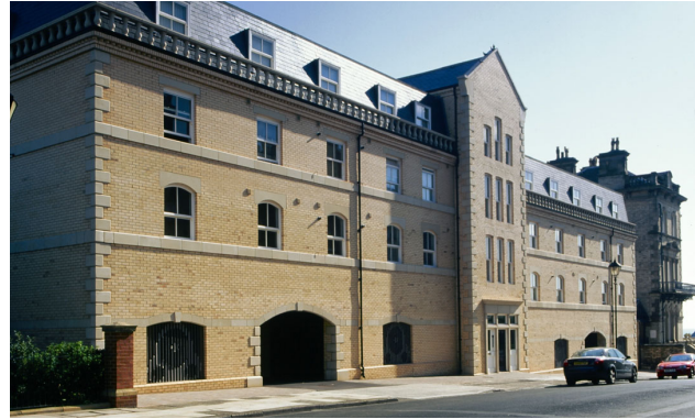
Fig 32. A relatively dense development at Saltburn, appropriate to context and housing a population likely to sustain local goods and services.
