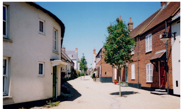
Fig 100. Physical measures such as trees in the calmed area, and doors opening onto the shared surface force traffic to slow.
