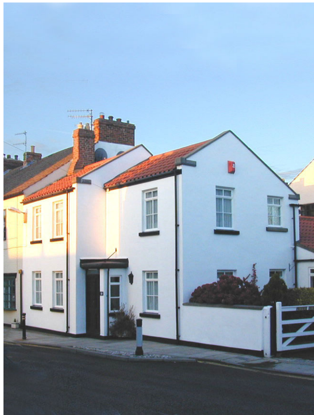
Fig 21. A successful extension in Guisborough. Its form subservient to the main dwelling and sympathetic in scale and materials.
