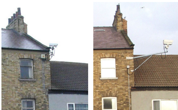
Fig 144-5. Wall mounted CCTV in Redcar. Reasonably subtle in 2003 but renewed at grotesque scale in 2004, undermining efforts to regenerate this terrace.
