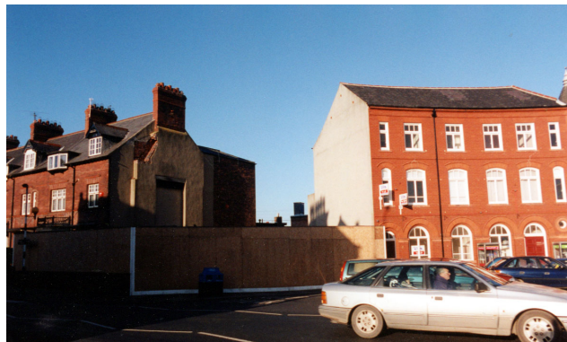
Fig 14. Windsor Road, Saltburn. A prominent corner site requiring careful bridging between three and 2 storey neighbours.
