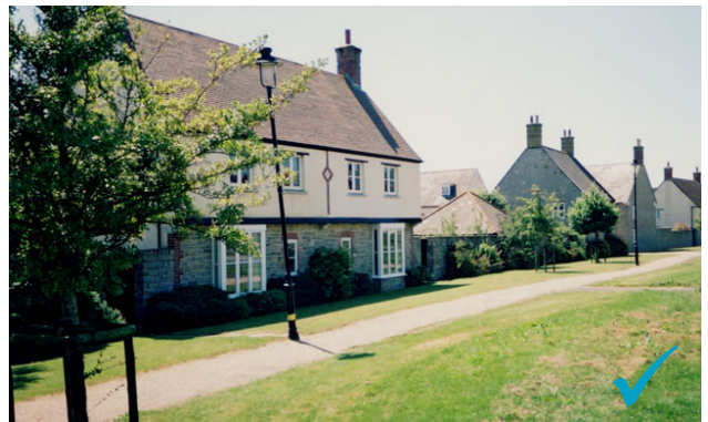
Fig 93. A new development where buildings actively face open space, reducing security risks and creating civic value.
