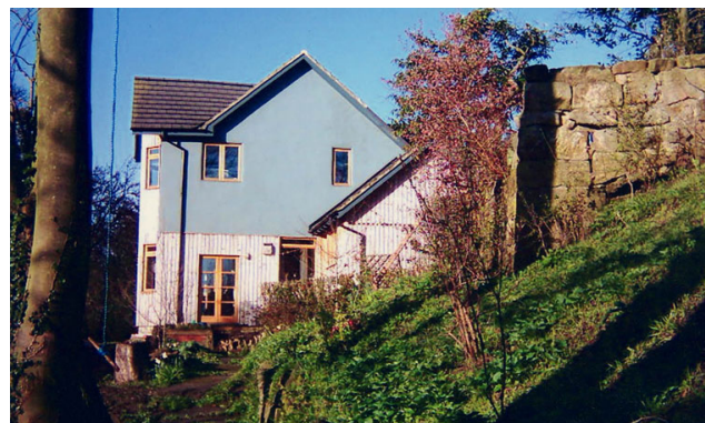
Fig 77. Timber framed dwelling at Loftus, one of whose roof pitches is a 'greenroof', providing habitat and additional insulation.
