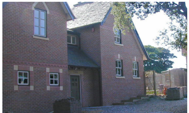
Fig 17. New building within the Conservation Area at Saltburn exhibiting sensitivity to context.
