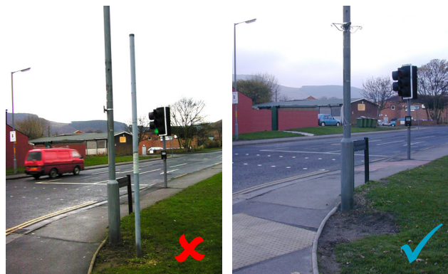
Fig 133-4. Left, defunct post. Clutters street and has been repeatedly weed-sprayed at base. Right, on removal.
