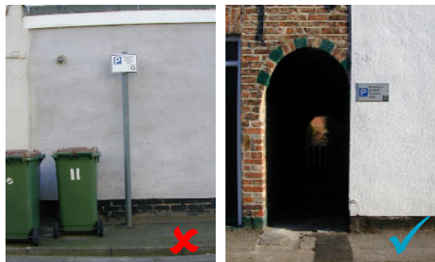
Fig 137-8. Where possible signs should be competently fixed to walls, reducing cost, clutter and maintenance requirements.
