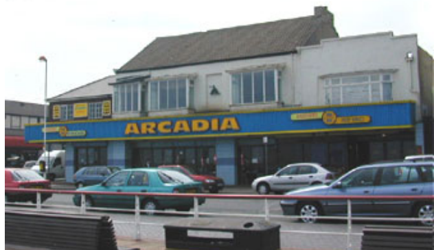
Fig 113. A crude, over large fascia that spans several buildings. Fascias should be divided up to relate to each 'design unit'.
