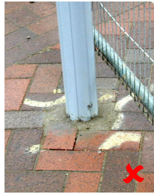
Fig 124. A crudely installed post and an unsafe and poorly installed barrier at Redcar.
