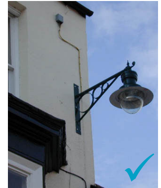
Fig 141-2. Where possible CCTV, signs and lighting should be wall-mounted. To the left the view through Regent Walk is marred by superfluous lighting columns. Wall-mounted versions, as at Chaloner St above, would have required less maintenance and materials and would have created a less cluttered appearance.
