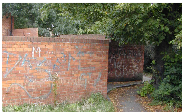
Fig 59. Detail of figure 60 showing footpath obscured by chicane in boundary wall. Lack of observation invites graffiti.
