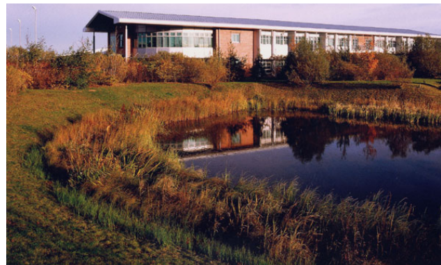
Fig. 155. Balancing ponds such as this at Kirkleatham can be used to moderate storm run off and replenish groundwater.
