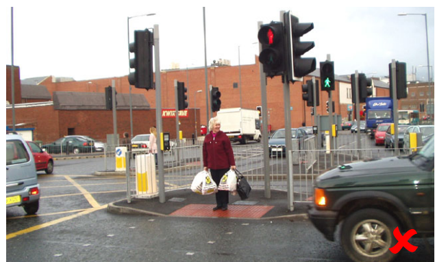
Fig 90. Recent pedestrian-unfriendly development, with buildings turning their backs on the street. Extensive engineering works place the pedestrian at a disadvantage over cars, compelled to take a tortuous route through barriers.
