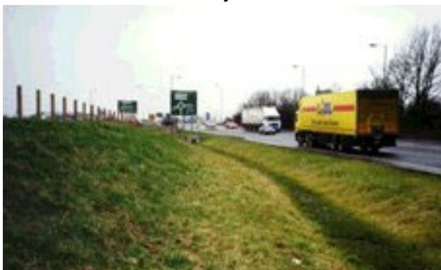
Fig 156. Swales and ditches can often be used on Highway schemes more cost effectively than piped drainage.
