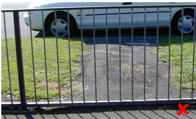
Fig 139. Pedestrian barrier at Glenside. The tarmac path it makes redundant has been left by oversight or thoughtlessness.
