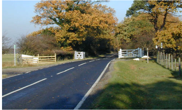
Fig 146. Approach to Liverton Village. Distinctive barrier and cattle grid emphasise rurality yet simultaneously calm traffic.
