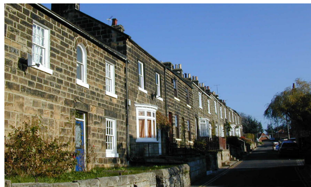
Fig 27. Stone terraces in Loftus, typical of East Cleveland and evidently durable and popular places to live.
