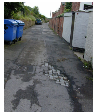
Fig.120-1. Scoria blocks, cast from furnace slag, remain in many back roads and alleyways, testimony to their durability.
