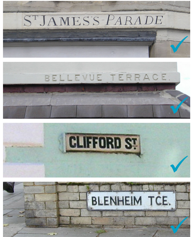
Fig 115. Integral name plates. Practically immune from vandalism and conveying quality and permanence. An appropriate fixing method will avoid any damage to the structure.
