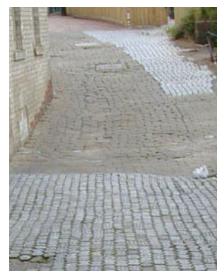
Fig 122-3. High quality scoria and expensive sandstone and brick setts at Loftus, concealed beneath tarmac.
