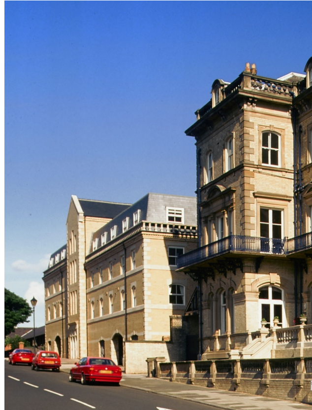
Fig 50. An infill development Dundas Street, Saltburn, responding to the scale of its exuberant neighbour the Zetland Hotel.
