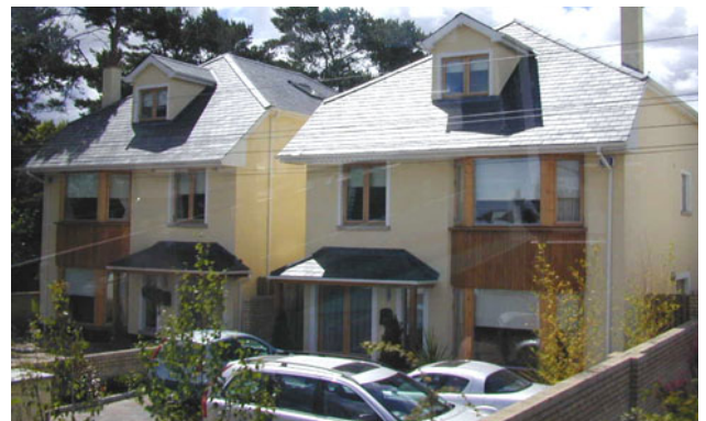
Fig 37. Use of attic space enhances available living space and in this instance adds interest to roof. Malahide, County Dublin.
