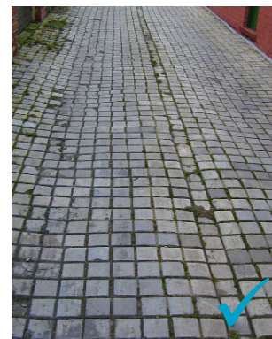
Fig.120-1. Scoria blocks, cast from furnace slag, remain in many back roads and alleyways, testimony to their durability.
