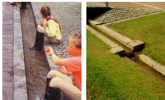
Fig. 157-8. New developments, as at Upton, Northampton, can incorporate SUDS schemes as key landscape elements.
