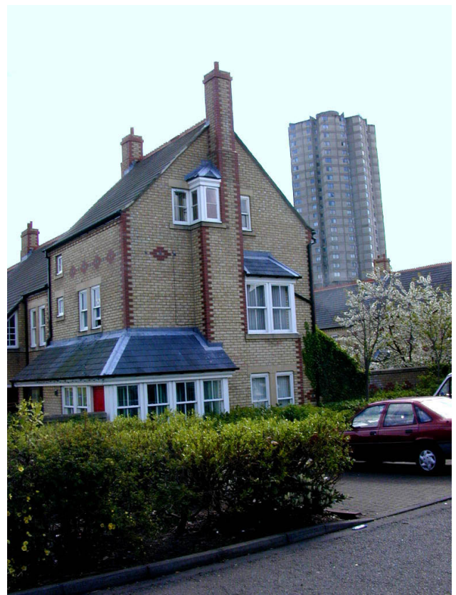
Fig 65. Here parking is well overlooked by windows which enliven a gable end.
