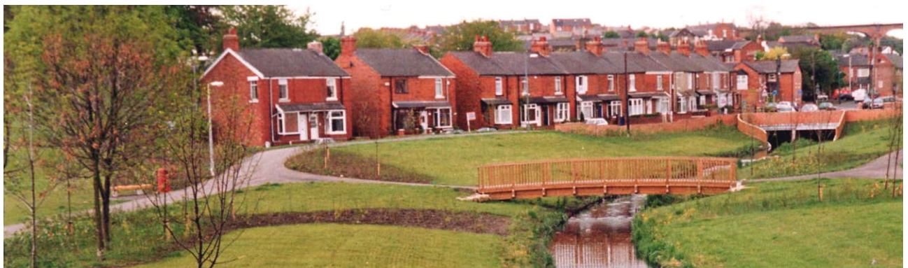
Fig 163. In a 1990's initiative, the site was remodelled to bring the watercourse back to the heart of the town. Culverts were removed and the Burn was restored to a graded natural channel, creating a significant townscape asset.
