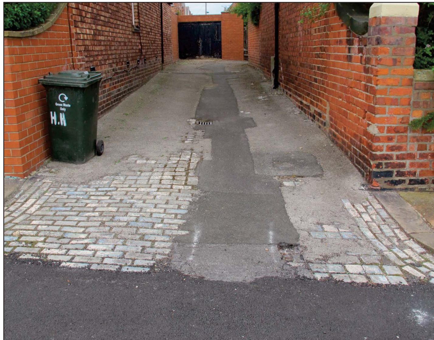
Patch repairs over original scoria block surfacing
