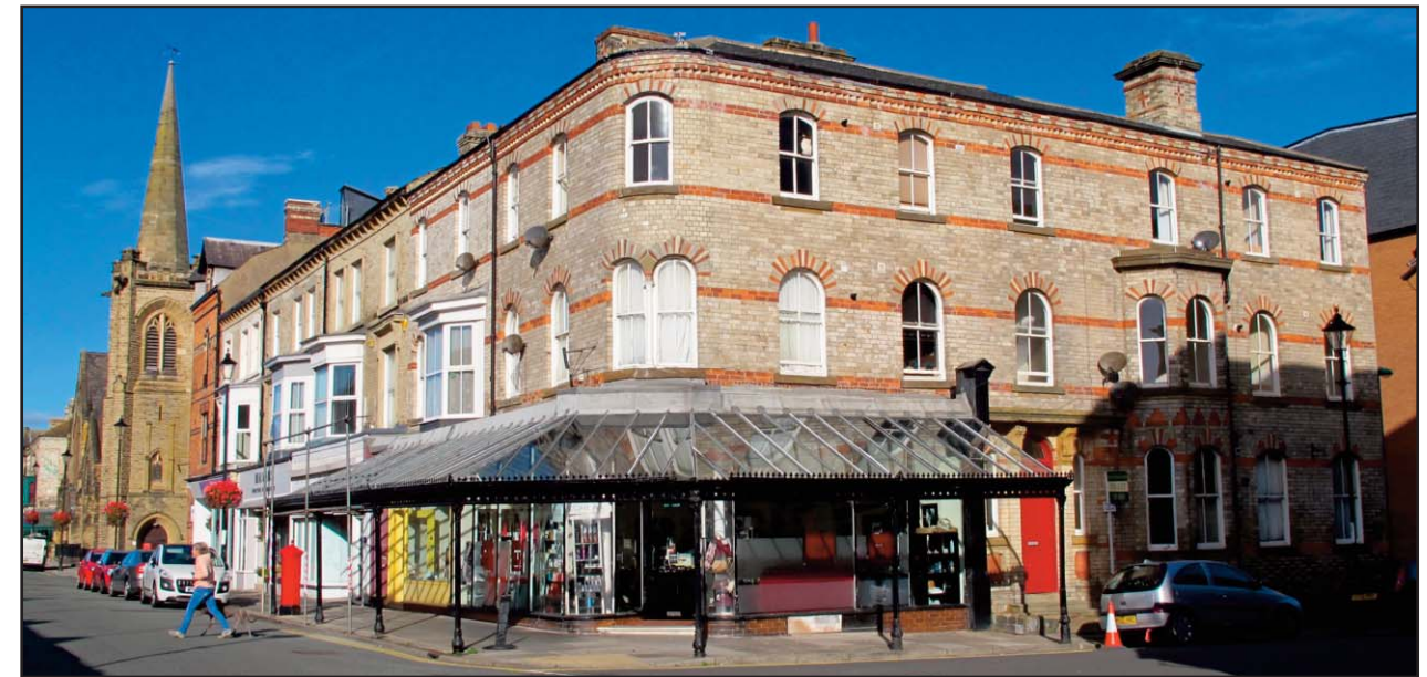
Historic cast iron canopy on Milton Street
