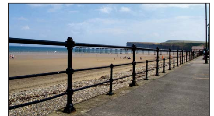
Cast iron railings on the foreshore
