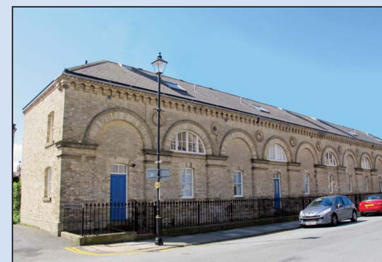
The loss of chimney stacks damages the character of a terrace*
