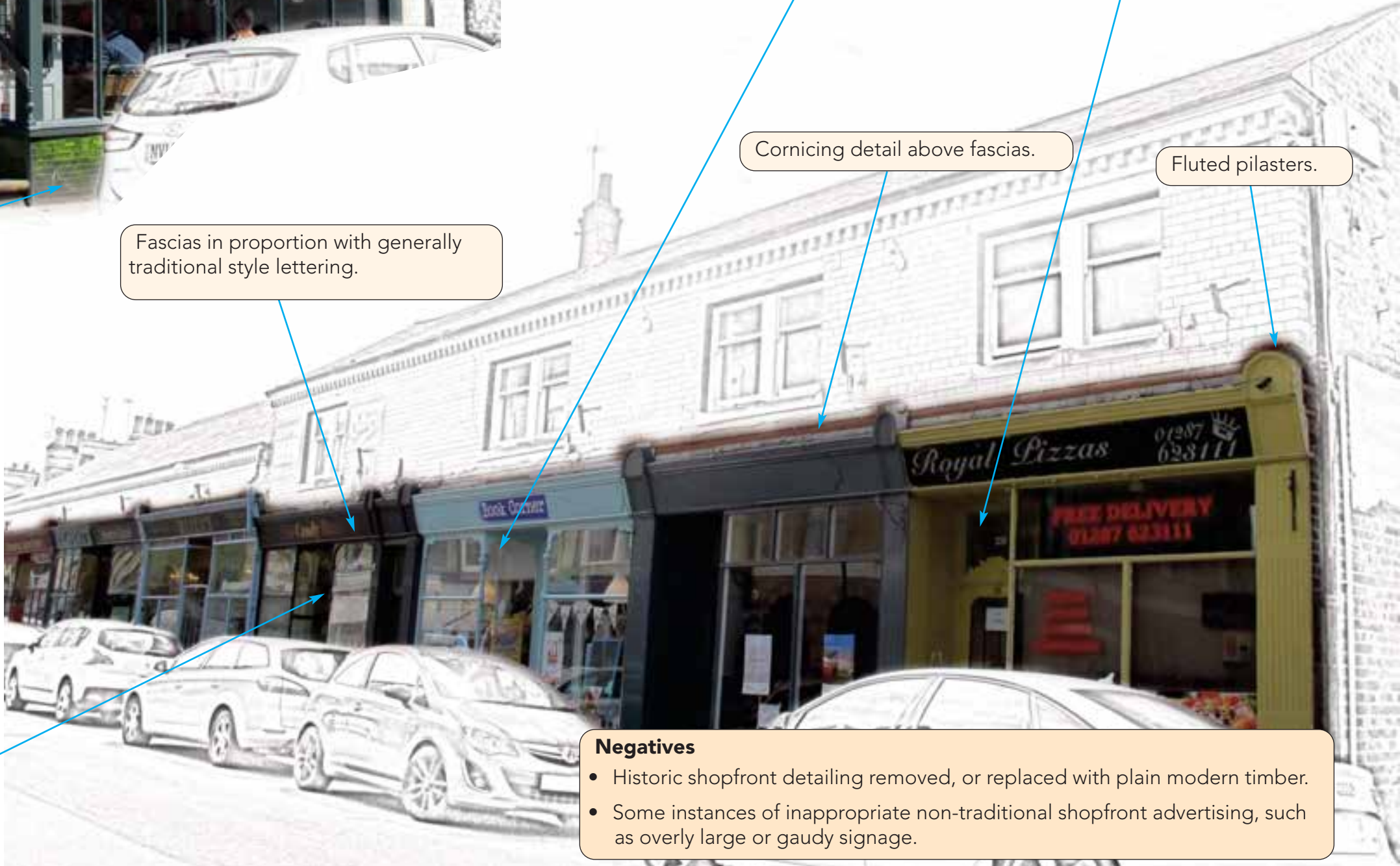
Stall riser matches facing materials. Others are frequently timber or sometimes glazed tiles.
