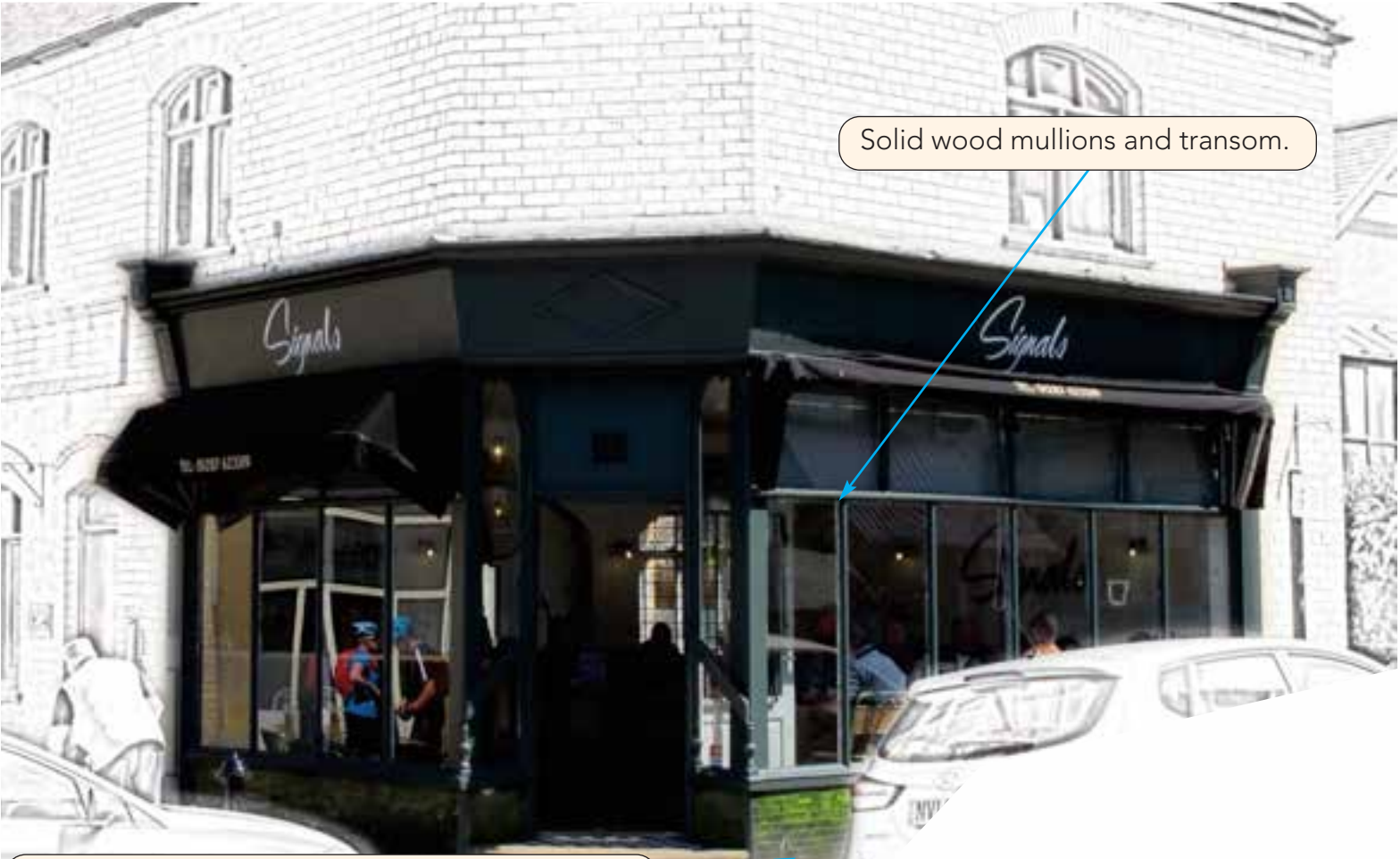
Stall riser matches facing materials. Others are frequently timber or sometimes glazed tiles.
