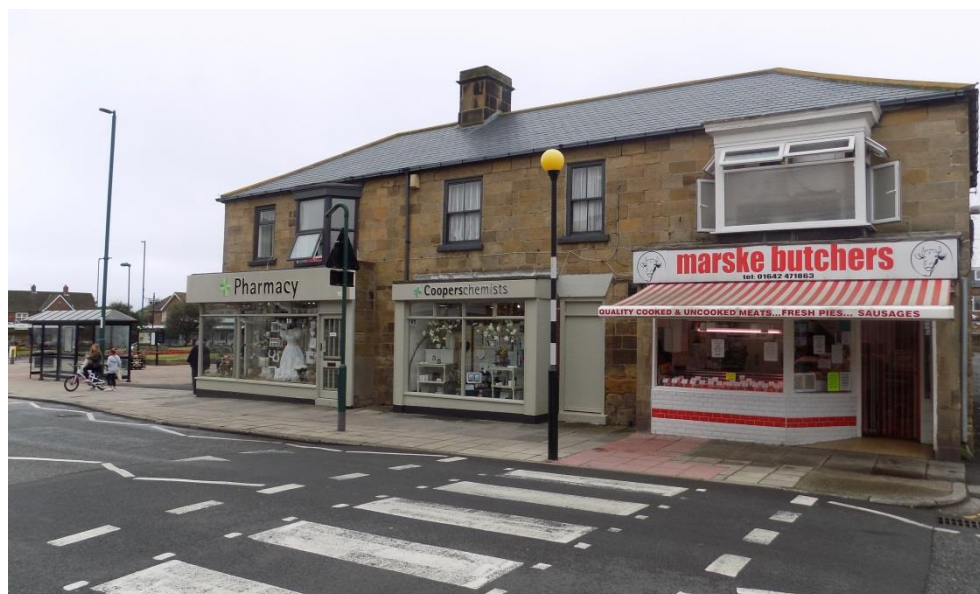
Figure 5.15 High Street, Marske District Centre
