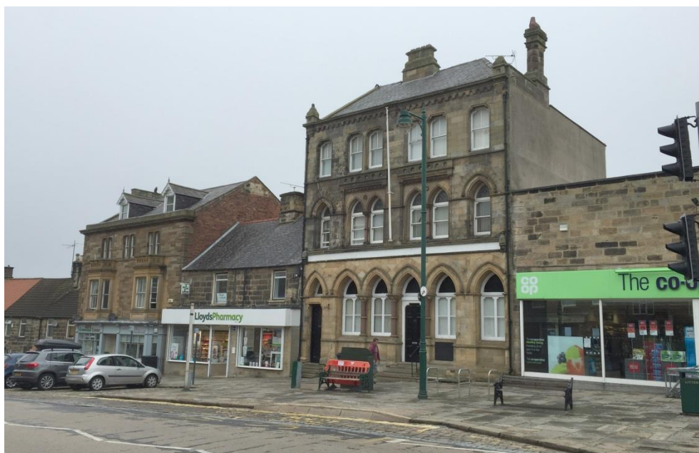
Figure 5.17 High Street, Loftus District Centre
