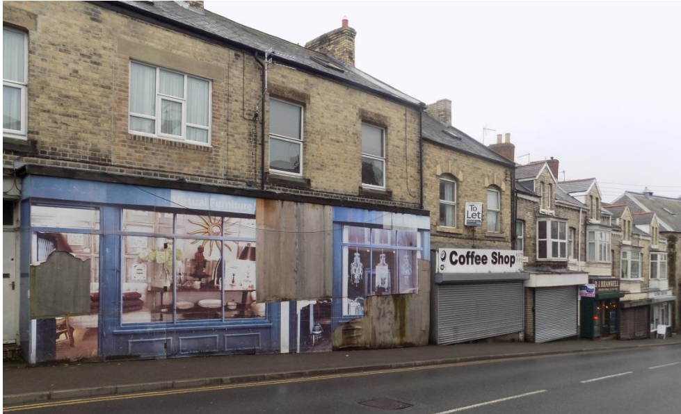
Figure 5.18 Zetland Road, Loftus District Centre
